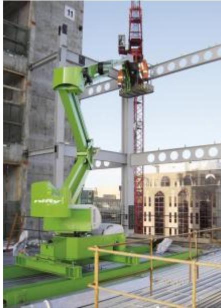
**Photograph 8** A deck mounted boom (Source – [www.niftylift.com](http://www.niftylift.com))
