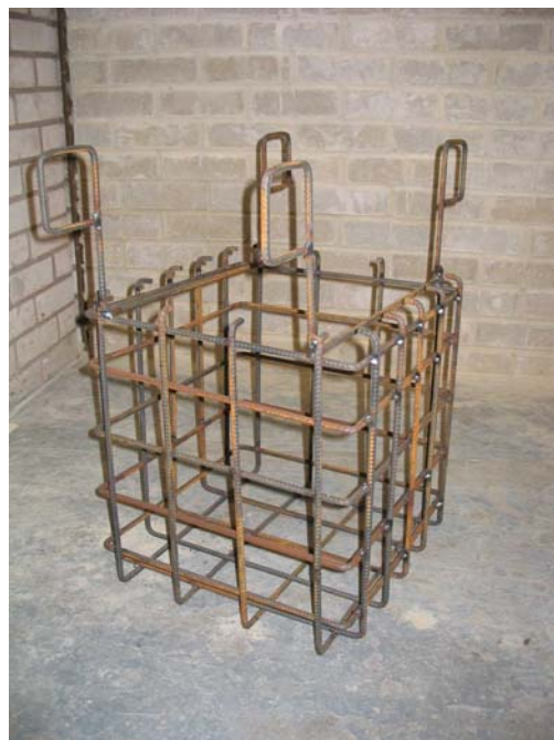
Figure 4: Lightly tied reinforcing steel rods
