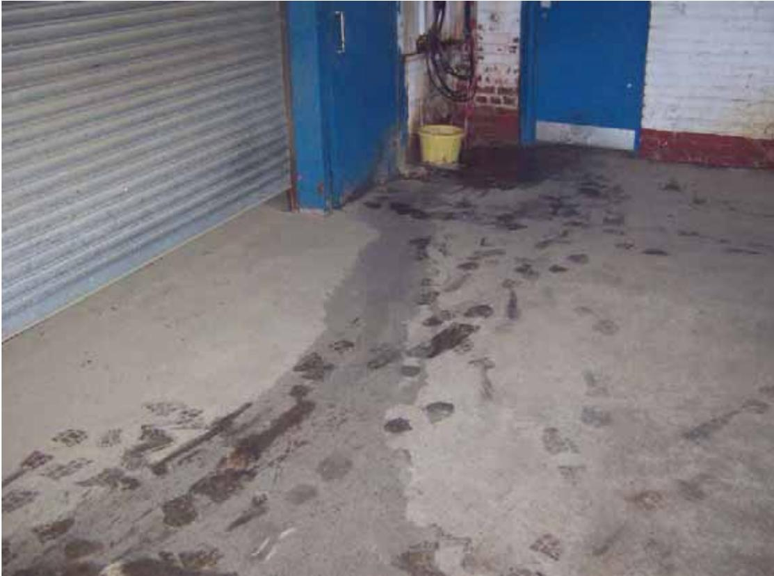
**Floor Type:** Powerfloated concrete with dry shake hardner
