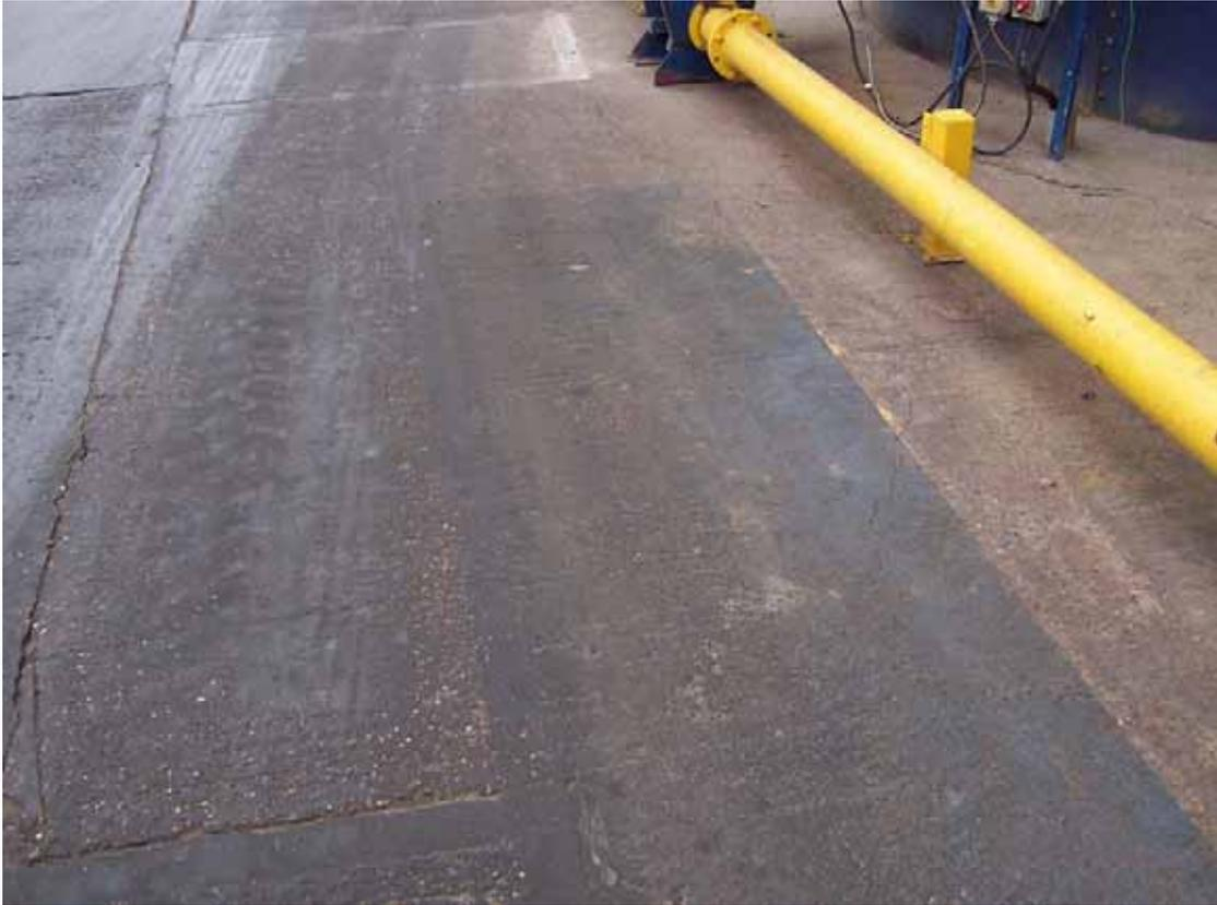
**Floor Type:** Concrete With Epoxy / Aggregate Coating
