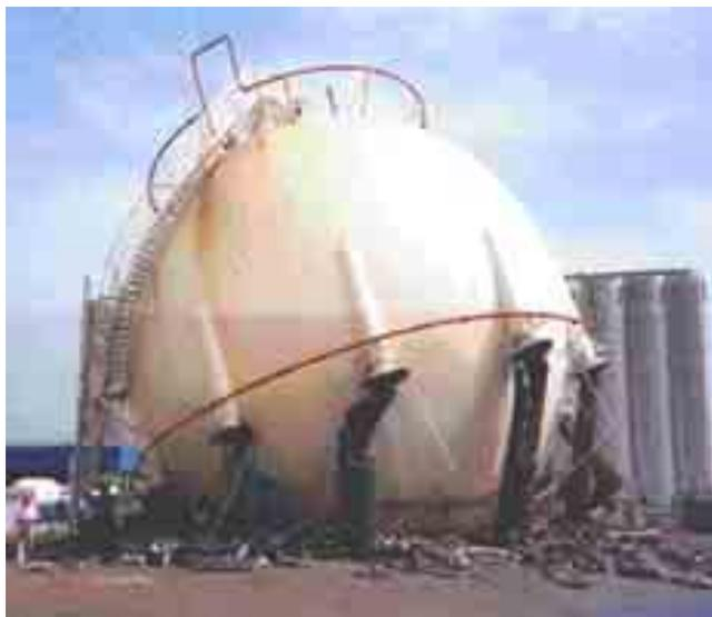
This storage sphere collapsed because one leg became severely corroded and could not carry the weight. A catastrophic failure was narrowly avoided. The lesson here is that supporting structures, although not pressure containing, are part of the system safety and need to be properly protected, managed and inspected (See Section 1.4.1 & 1.4.3).
