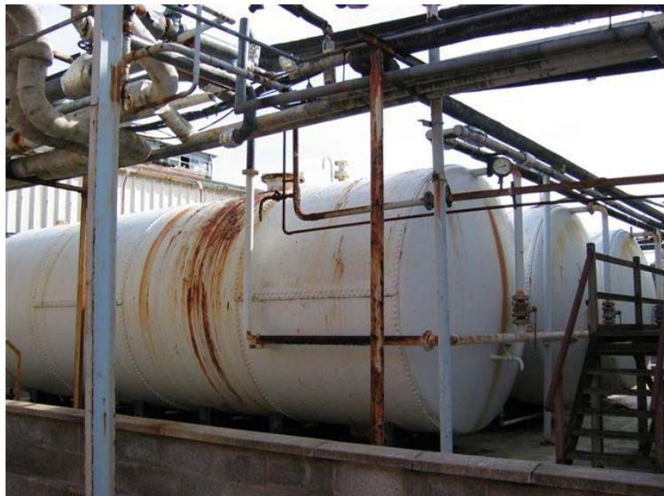
**THESE PRE-WAR RIVETED PRESSURE VESSELS REMAINED IN GOOD CONDITION AND SUCCESSFULLY OPERATED IN SERVICE UNTIL THE 1990'S**
