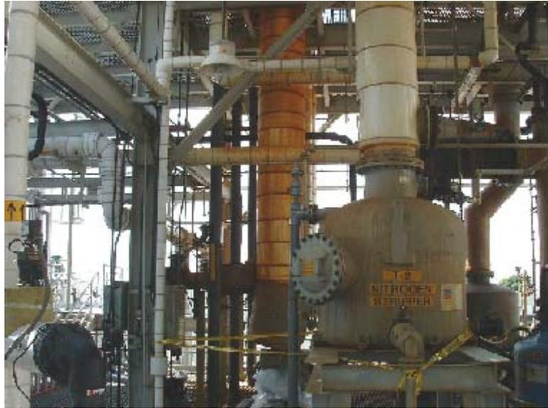
**THIS PLANT WAS ONLY ABOUT 5 YEARS OLD, BUT DUE TO POOR MAINTENANCE WAS STAINED IN MANY LOCATIONS FROM ACID SEEPAGE. THIS MADE IT HARD TO INSPECT AND TO KNOW HOW IT WAS AGEING.**
