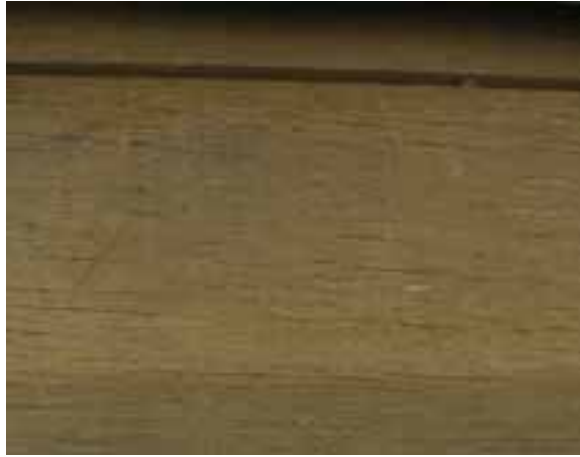
Figure 17 - Wooden Planks Surface
