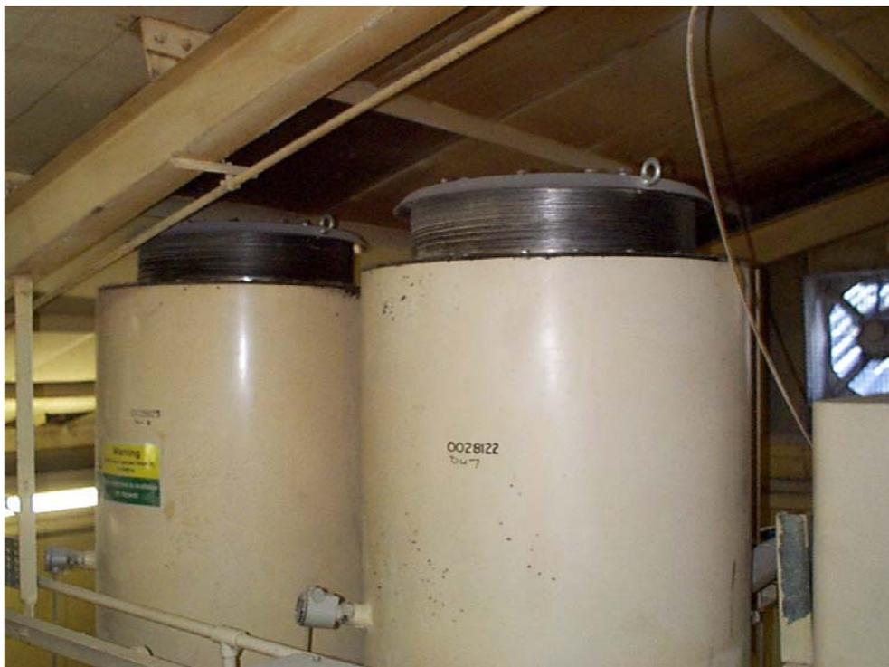
**Figure 16: Flameless venting devices fitted to flour bins**
