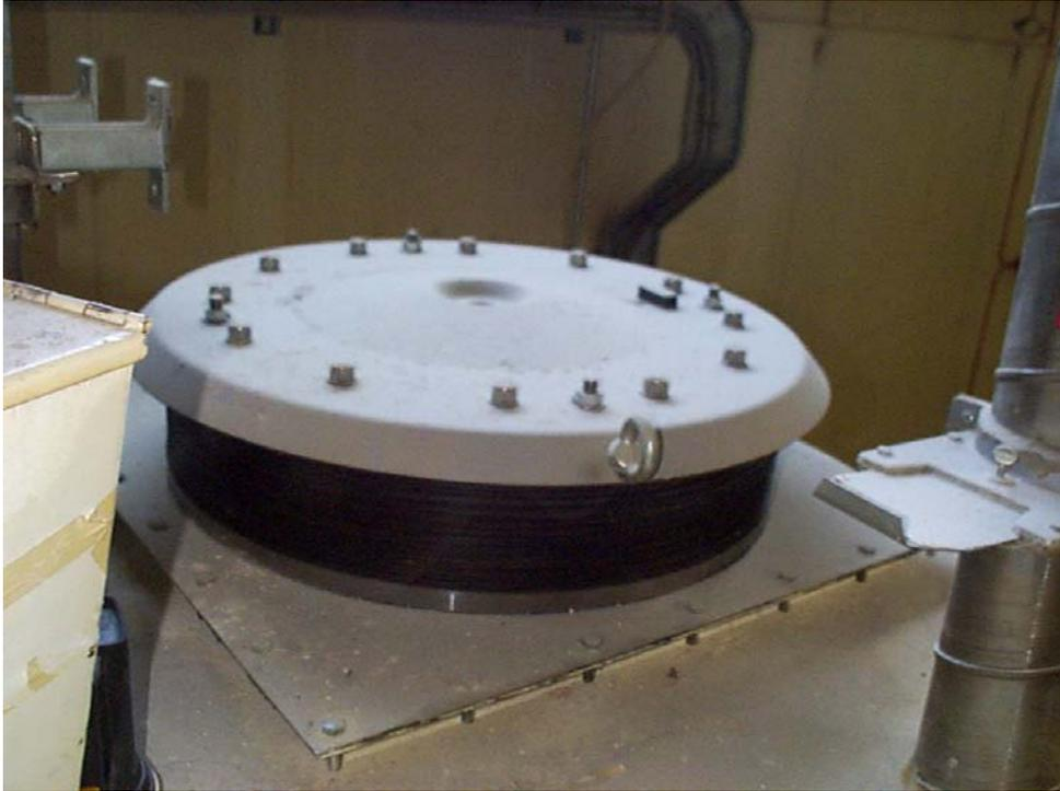
**Figure 15: Flameless venting device fitted to a batch bin**
