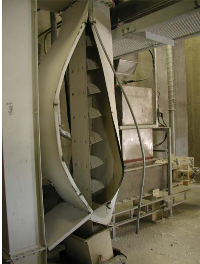
**Figure 11: Ruptured elevator casing**
