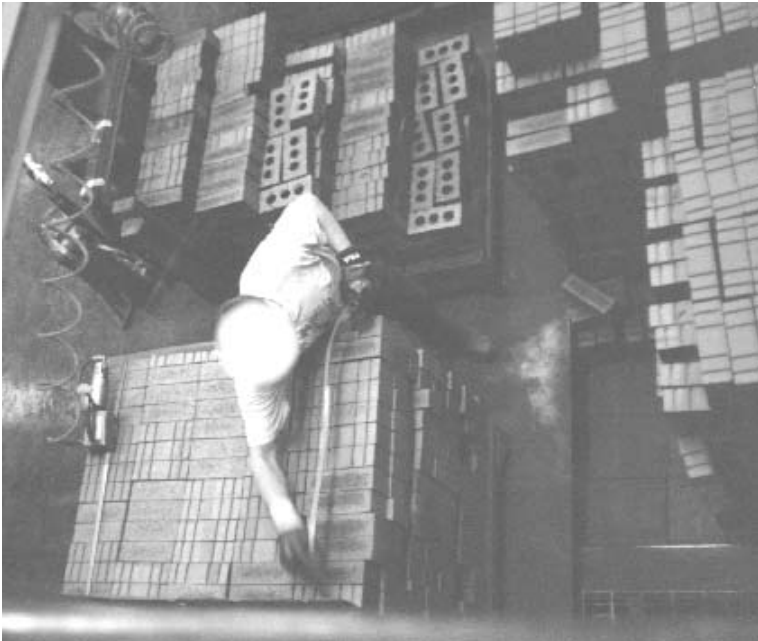
Figure 3: Hand strapping of bricks with an air powered strapping tool.
