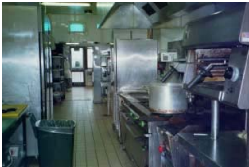
Position of the monitor in some of the surveyed kitchens
