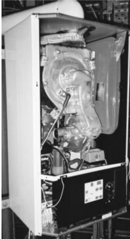
**Figure 4 - Ecomax - photograph of boiler (air inlet pipe removed)**
