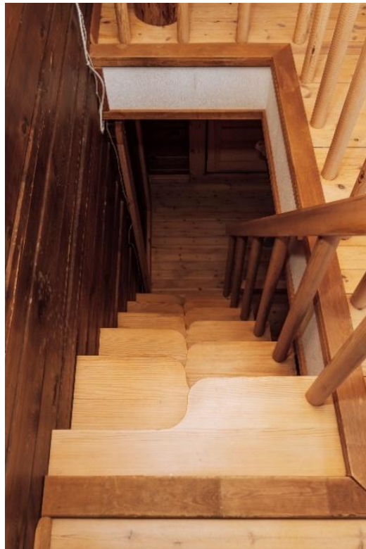
Figure 20. Alternating tread stairs (source: Getty Images, under HSE licence. Images are for illustration purposes only and do not necessarily represent compliance or good practice.)
