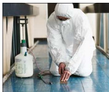
Spray at low pressure; high-pressure spray could disturb fibres from asbestos paper under these tiles
