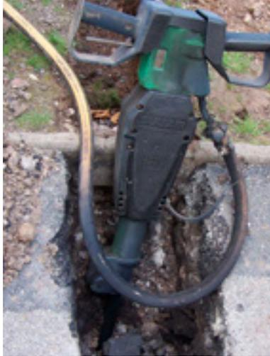
This charred breaker has struck an 11KV cable in a shallow trench
