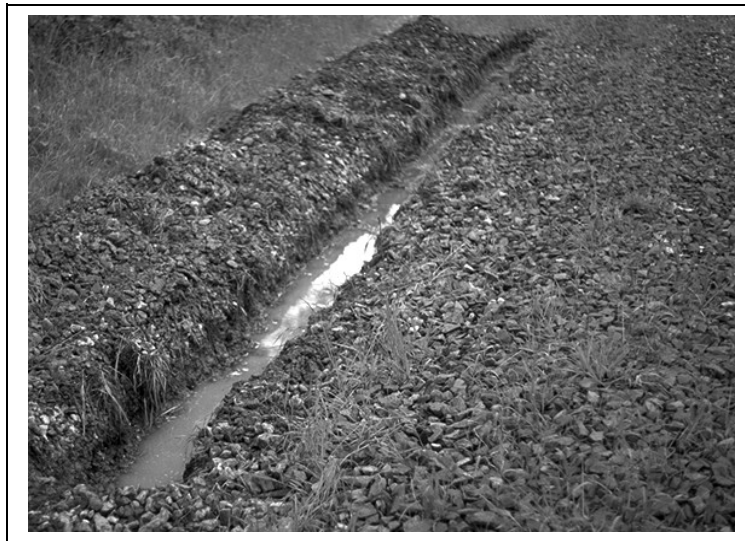
Plate 3: One of the sampling trenches, viewed from the ballast side
