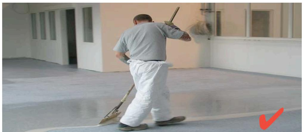
**Figure 7** With the help of a long-handled spreader, an adequate safe working distance has been applied, reducing the likelihood of contact with the coating. It reduces the potential for back problems too
