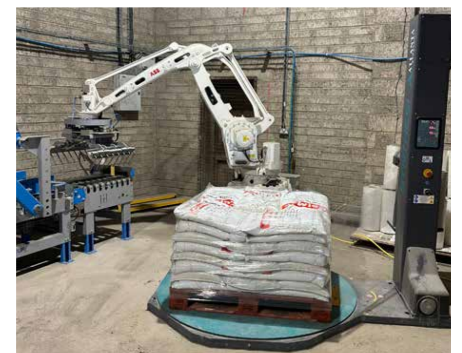
Robotic arm and automatic pallet wrapper
