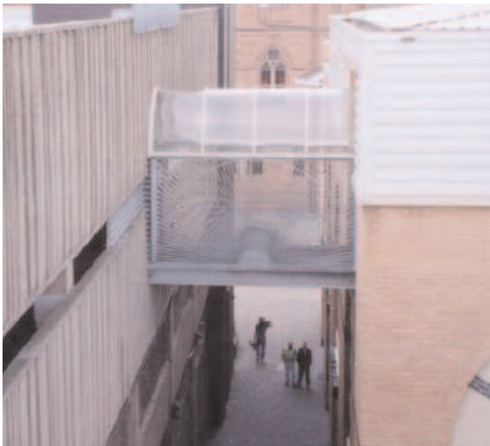
Figure 1 The alleyway next to the Forum 28 building
