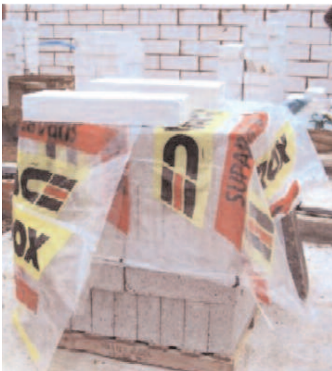
Figure 1 Blocks covered by polythene sheeting to keep them dry
