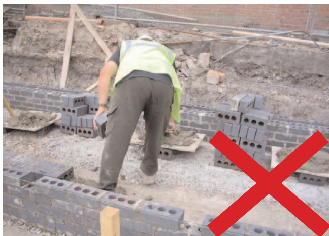
Figure 1 Bending to trowel mortar and lay bricks at ground level
