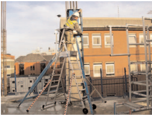
Figure 1 Podium steps in use
