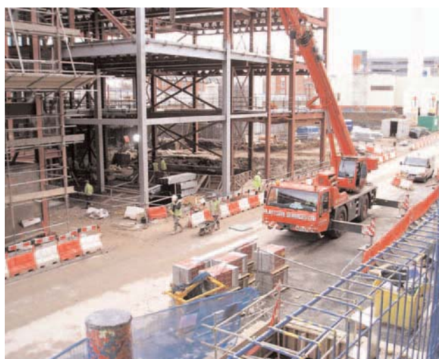
Figure 3 Work on the site
