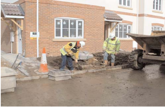
Figure 2 Workers digging after the issue of a permit to dig
