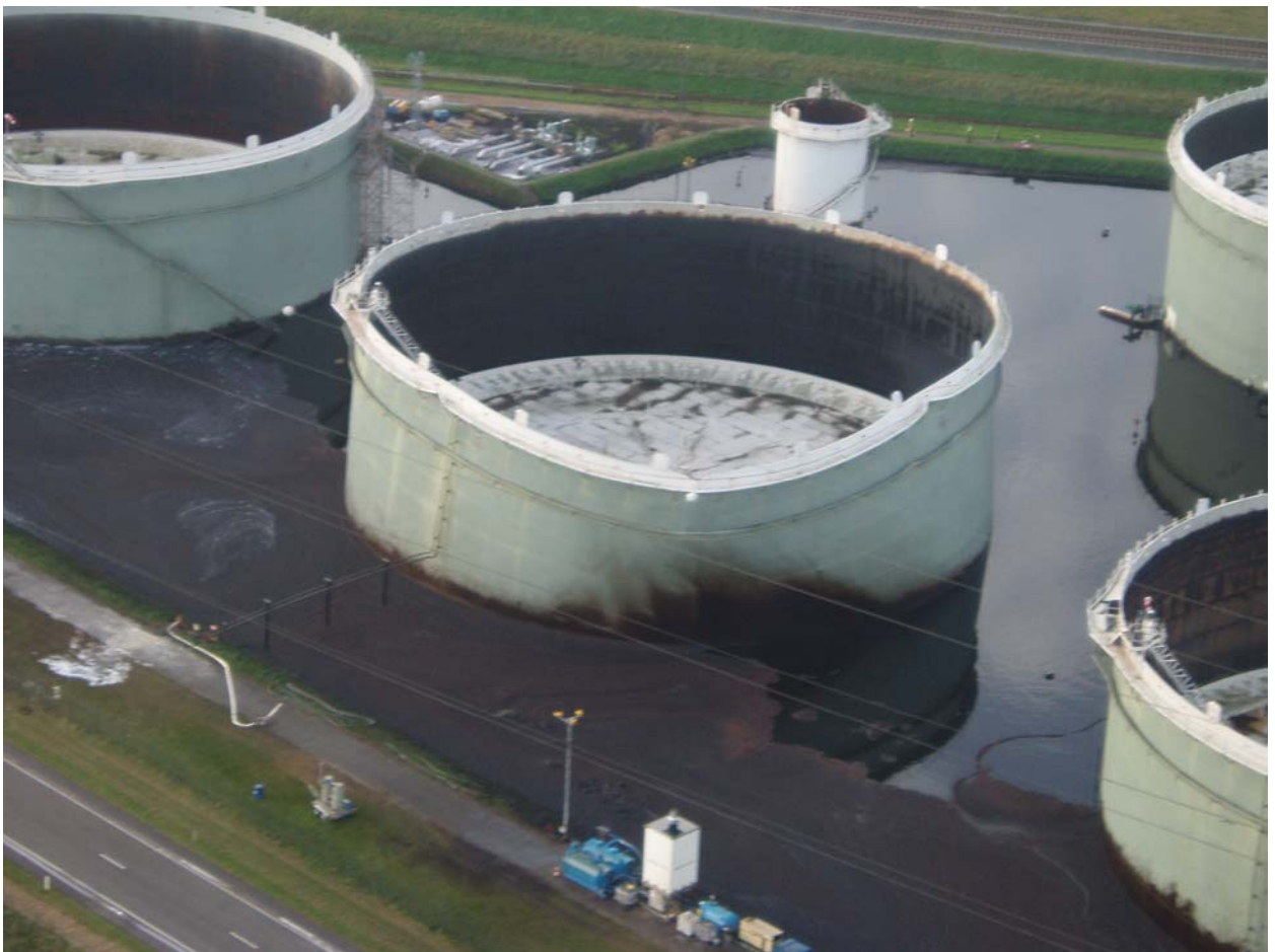
Figure 2: Picture of the situation in the bund the morning after the major accident
