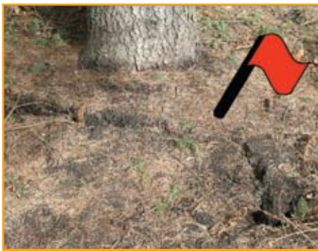
Tilted root flare of a spruce tree – A raised root flare and cracks in the soil indicate primary tipping failure. These trees may be very unstable.
