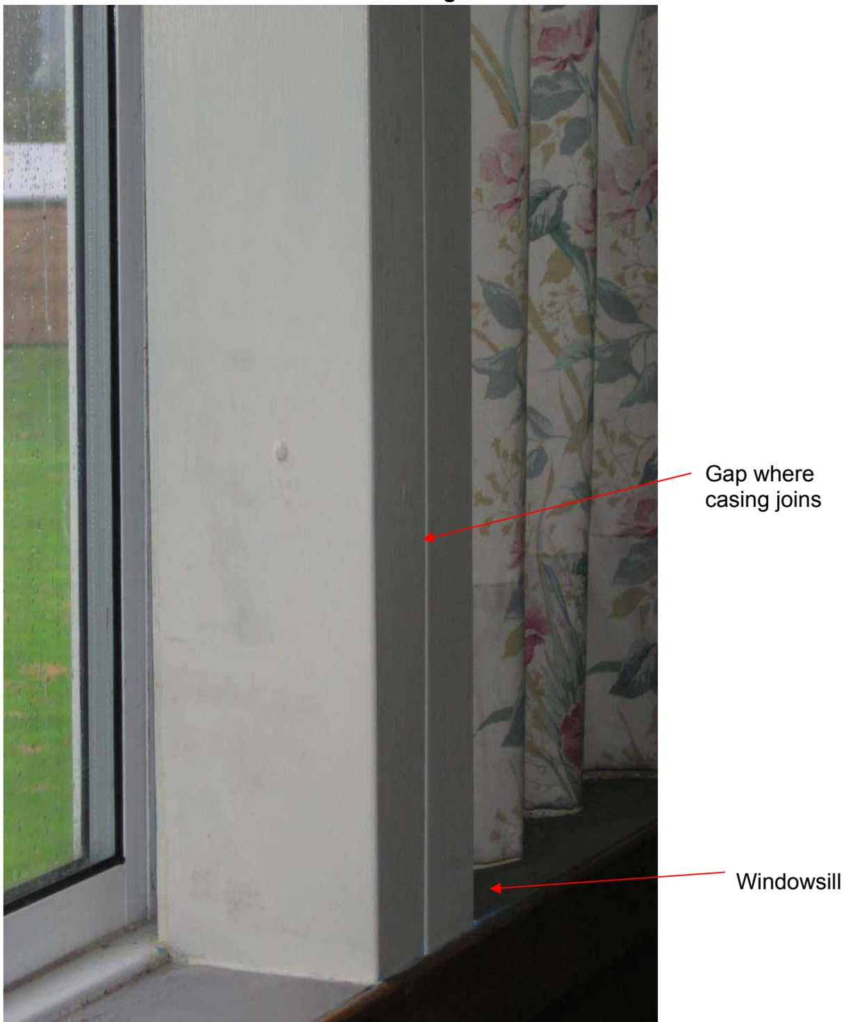
**Figure 3: Window column with half the section of casing removed – revealing the column and AIB**
