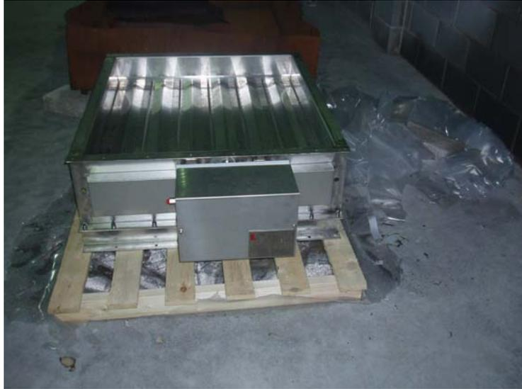
**Figure 8 A photograph of the fire damper as delivered. The damper is front face down with the actuator mechanism nearest the camera.**
