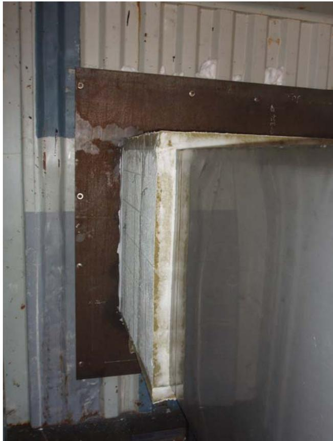
**Figure 17 A view of the insulation installed at the forward end of the ducting**
