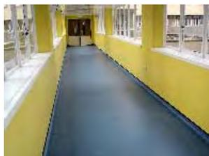
**Figure 18** New safety flooring on bridge link
