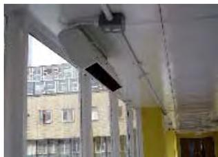
**Figure 19** Heaters to stop condensation
