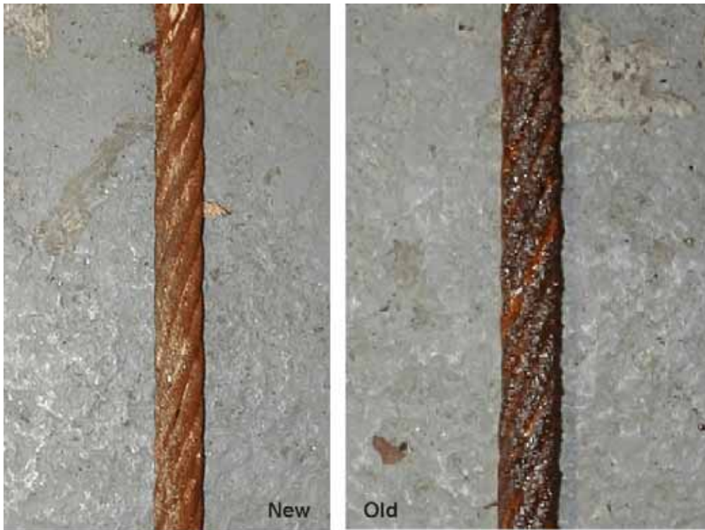
Figure 8 Rope samples after accelerated corrosion for 5 weeks
