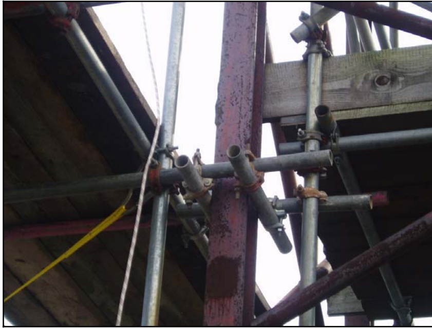
Figure 6 - As installed Box Tie
