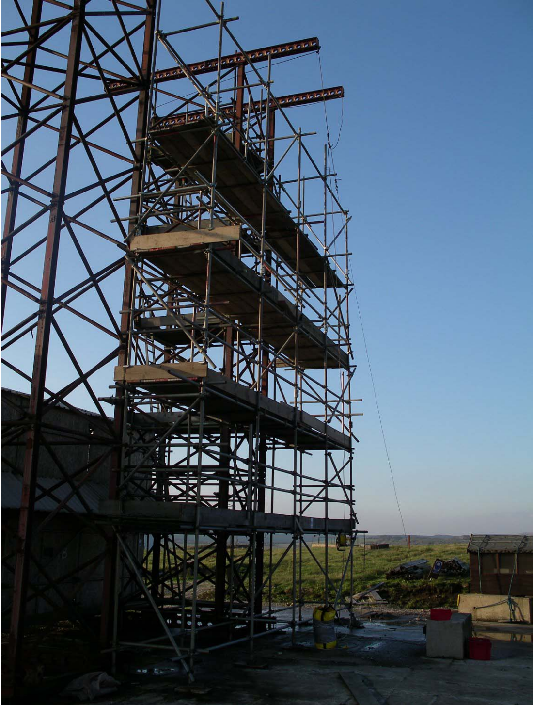
Figure 5 - Completed Experimental scaffold
