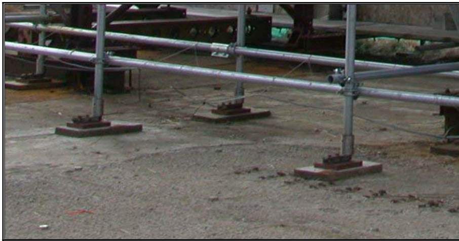
Figure 2 - Showing Base Loadcells
