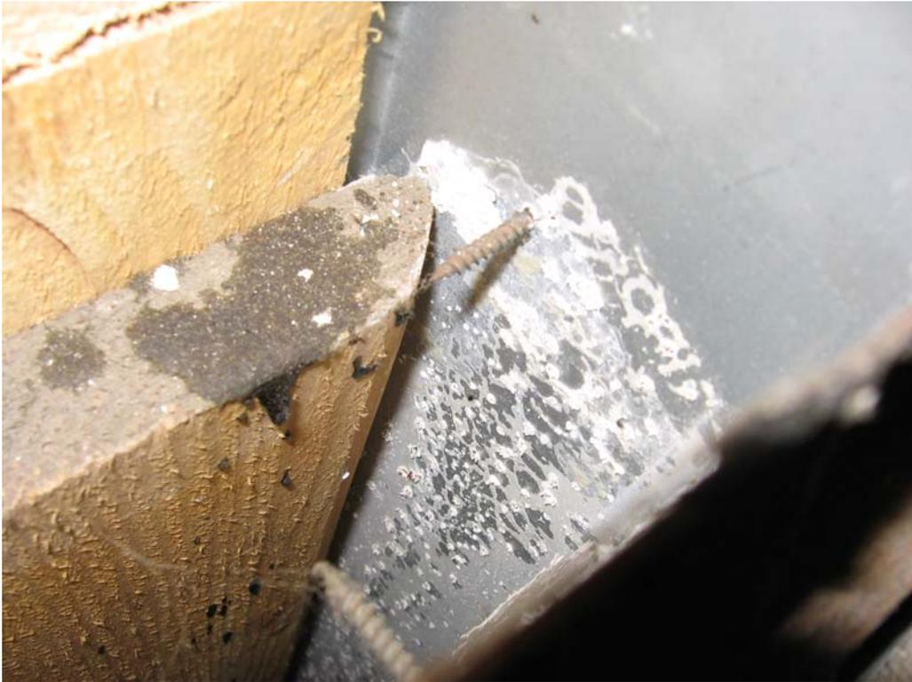
Figure 13: Example of asbestos debris from pieces of AIB that was glued onto the casing but had been torn off at some time. View down the column from above the suspended ceiling.
