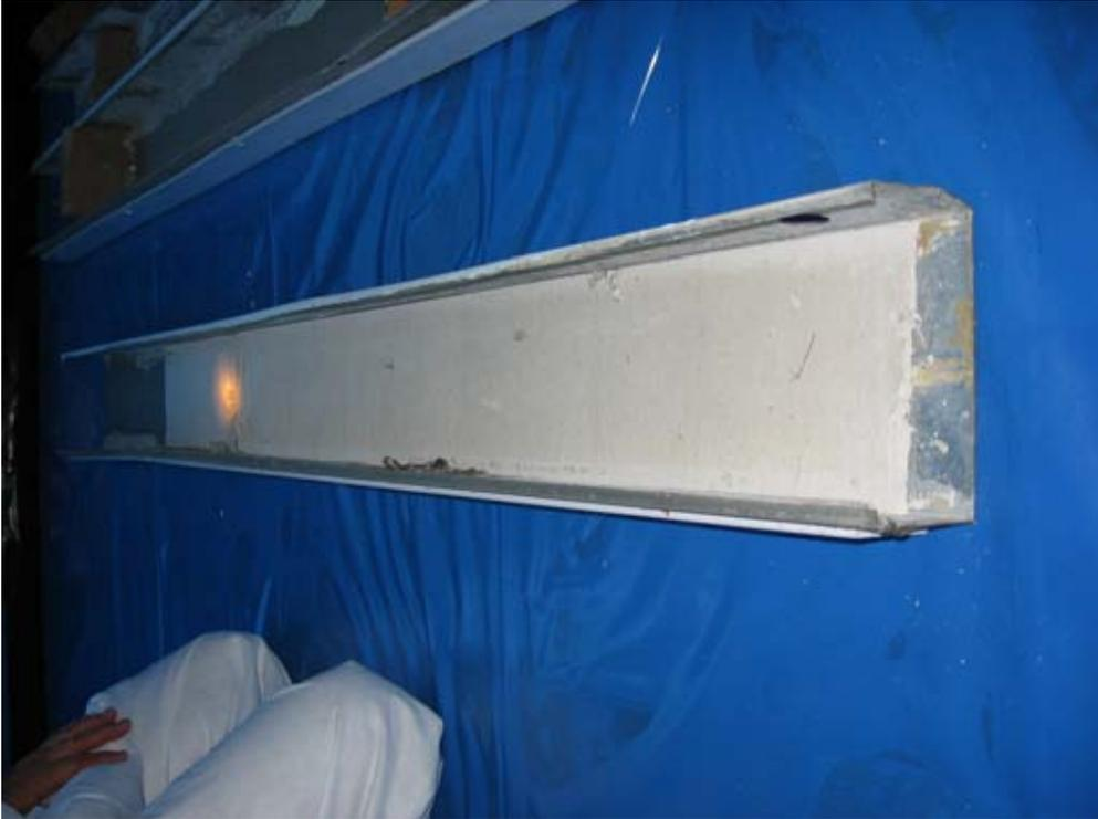
Figure 10: Example of a column casing with AIB attached to one side of the casing. The torch beam shows where the AIB has fractured due to a screw being placed into the casing. A hole is visible in the side of the casing and visible debris shows that friable material was present.
