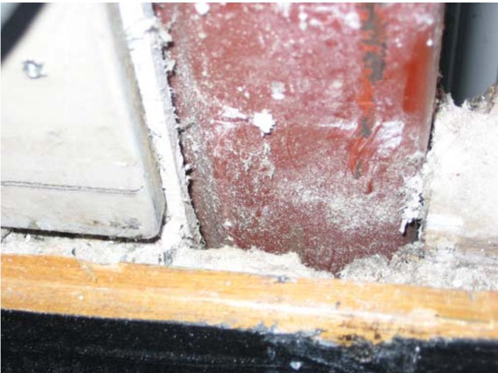
Figure 11: View of base of column from which the casing in figure 10 was removed. A large amount of friable AIB debris can be seen.
