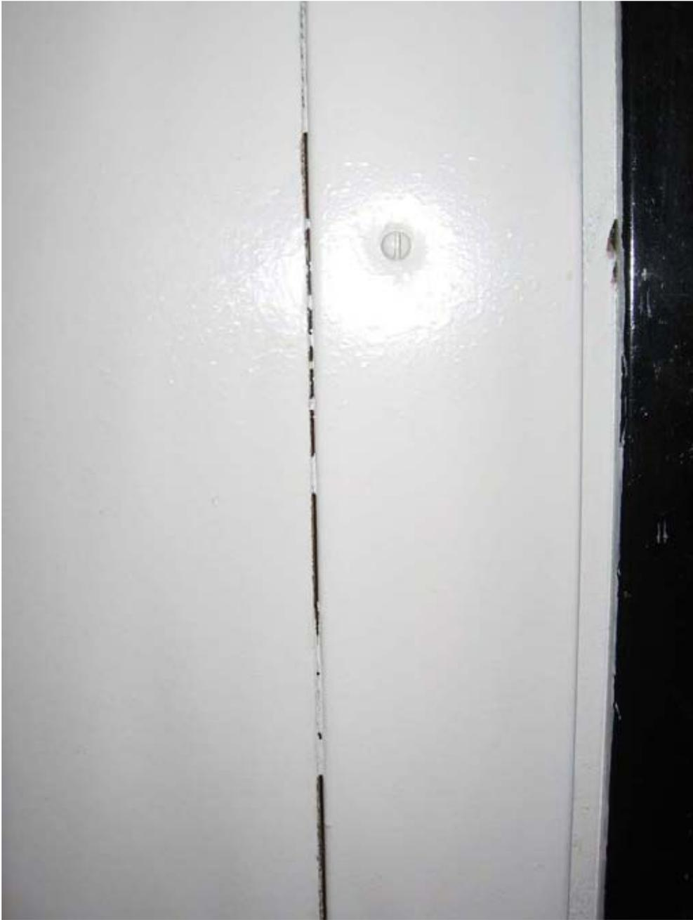
Figure 12: Example of a gap in the casing.
