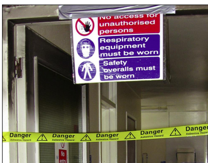
Make sure you restrict access
