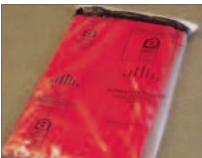
Double wrap the door in polythene sheeting with asbestos warning stickers
