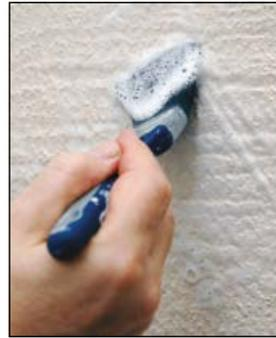
Paint sealant around the hole before you insert the screw. Use shadow vacuuming (if Class H vacuum available) to control dust when removing screws
