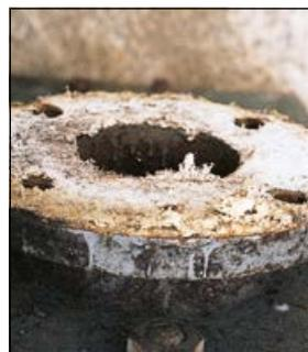
Gasket material left on a pipe flange
