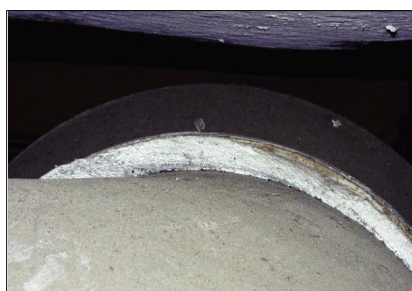
Joint packing on a flue
