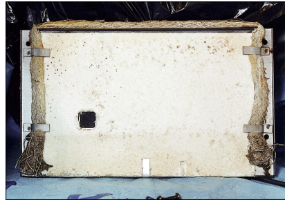
Some examples of rope seals found on boilers
