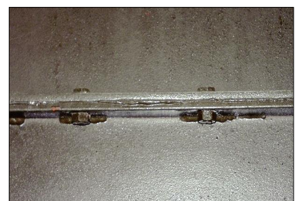
String gasket between metal sheets
