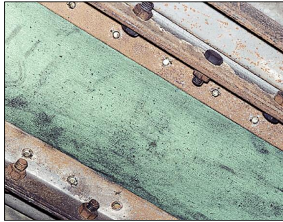
Riveted connector detail
