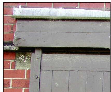
Built up bituminous roofing and bituminous asbestos fabric over a doorway
