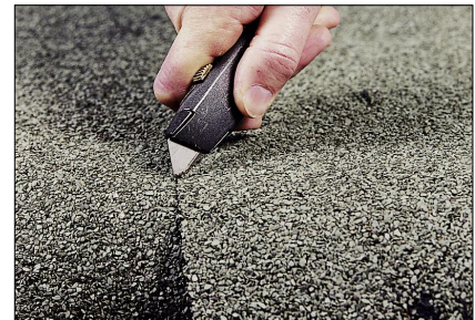
Cut and remove manageable sections
