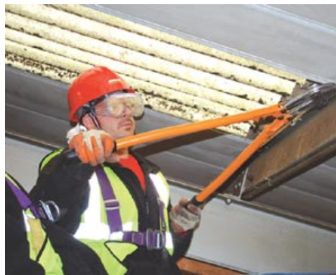
Removing hook bolts from existing sheet
