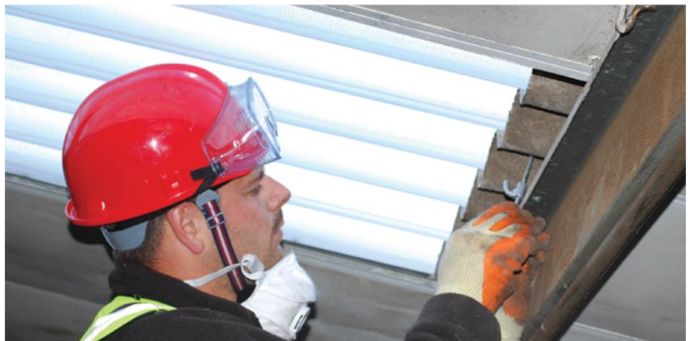
Securing fixings to newly installed sheet
