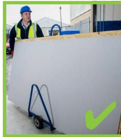
Stooping and twisting whilst moving panels cause huge strain on the body over time. A panel handling trolley allows better vision and one person can move several panels at once.
