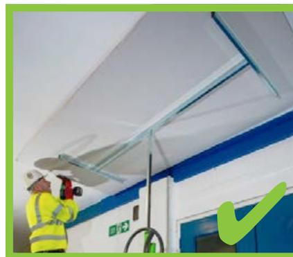
Fixing to ceilings is a common cause of strain for workers holding panels. Using a panel lifter allows one person to quickly fix panels with far better posture.
