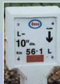
*Beware* of posts with brass studs (such as the post above) which have cables connecting to the pipeline below.
