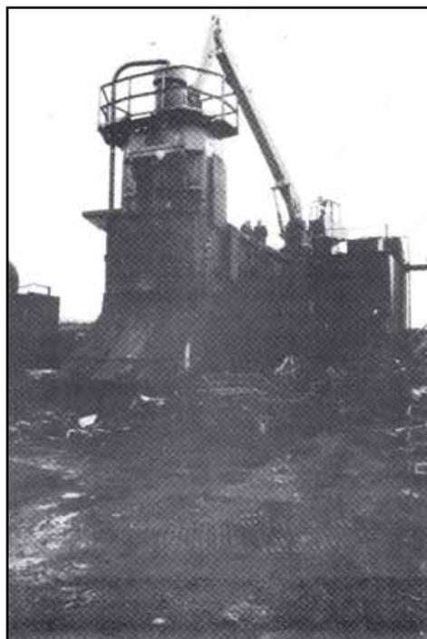
**Figure 4** Box Shears - view of exit chute from shears. Note protective metal shield to prevent cut scrap flying.
