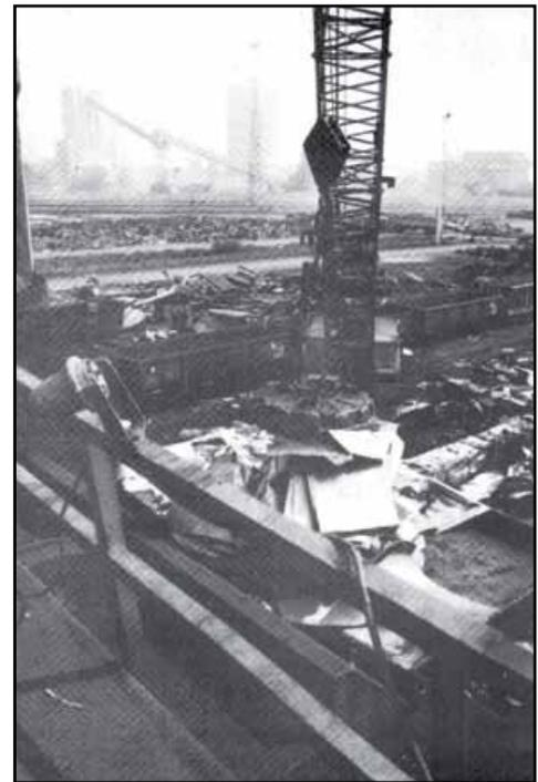
**Figure 2** Large mobile baler - loaded by crane and independently powered by diesel engine
