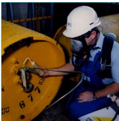
Testing for leaks following connection of the pigtail to the drum's gas take-off valve
