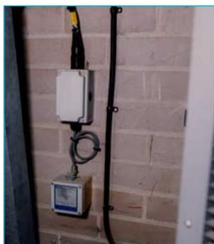
Chlorine detector located close to the fan inlet. The fan is activated by the low level alarm and deactivated by the high level alarm
