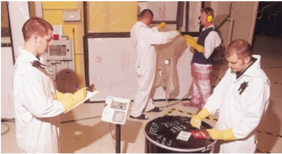
Packing waste from decommissioning the PUMA cell which had been used for criticality experiments.
