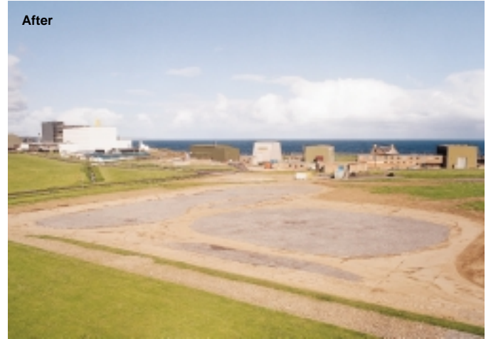
Compound with all buildings and soil removed.
