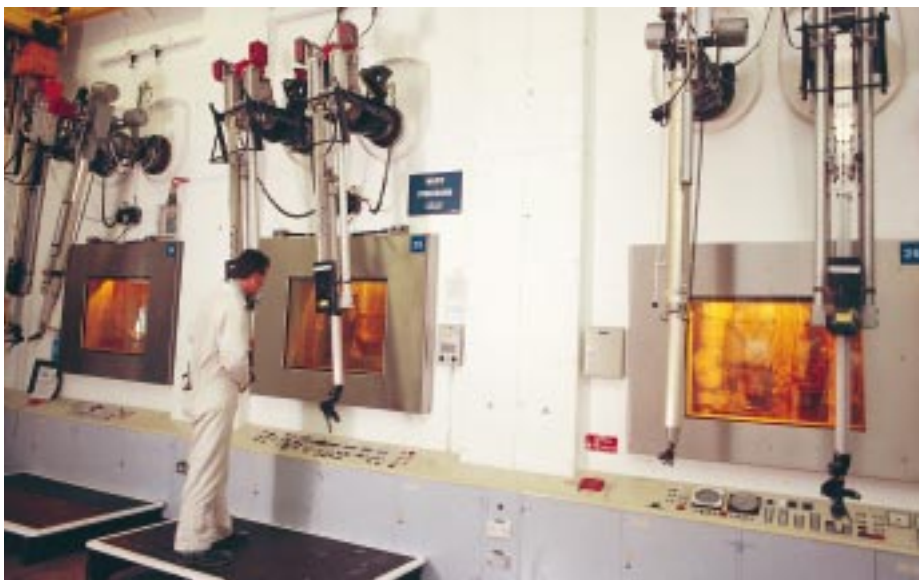
D2001 cell face after renovation
