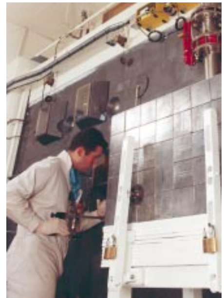
Lab 33 ventilation improvements (see text overleaf)
