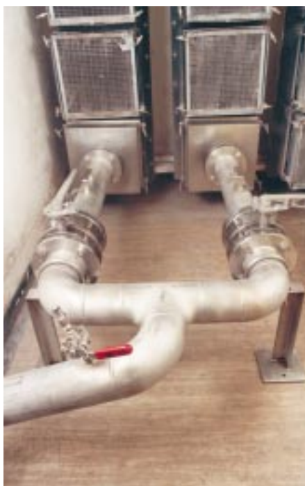
D9867 ventilation improvements
