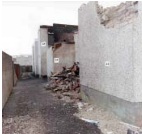
Figure 2 Path at front of 21 – 29 Linfield Street
