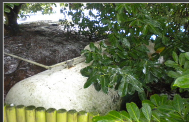
Tank in overgrowth
