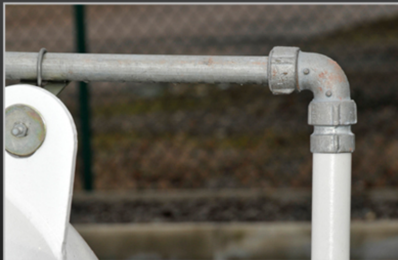
Polyethylene (PE) pipe enclosed in glass-reinforced plastic (GRP) sheath
