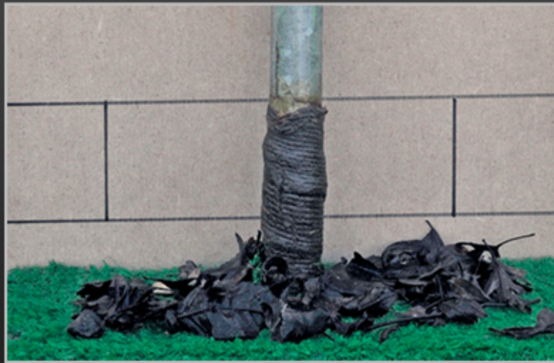
Pipe with Denso tape wrapped round its base
