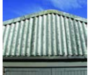
Asbestos cement panels
