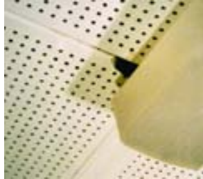
Asbestos insulating board ceiling tiles
