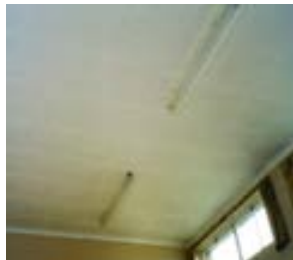
Asbestos insulating board panels
