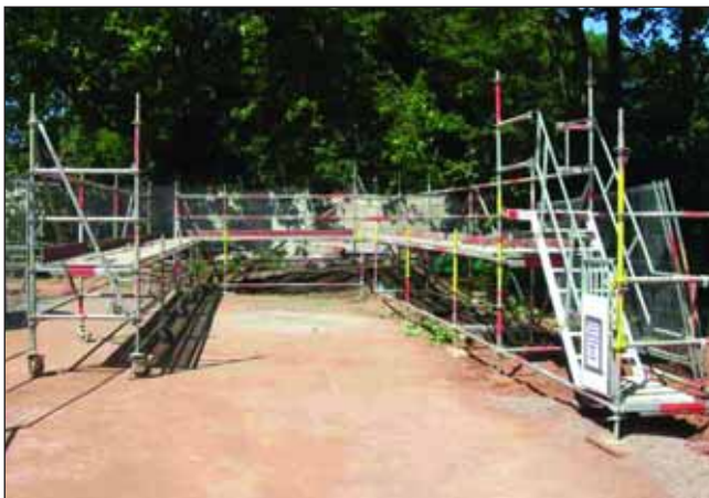
Figure 2 System scaffold unloading gantry
