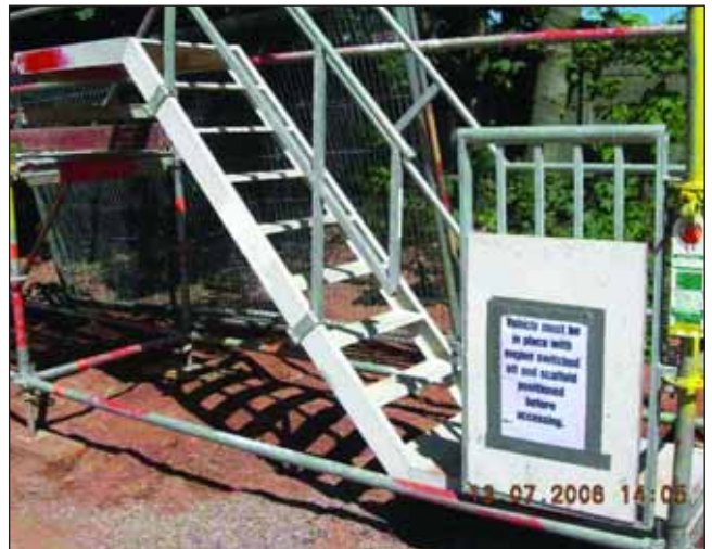
Figure 3 Safe stair access onto the scaffolding system
