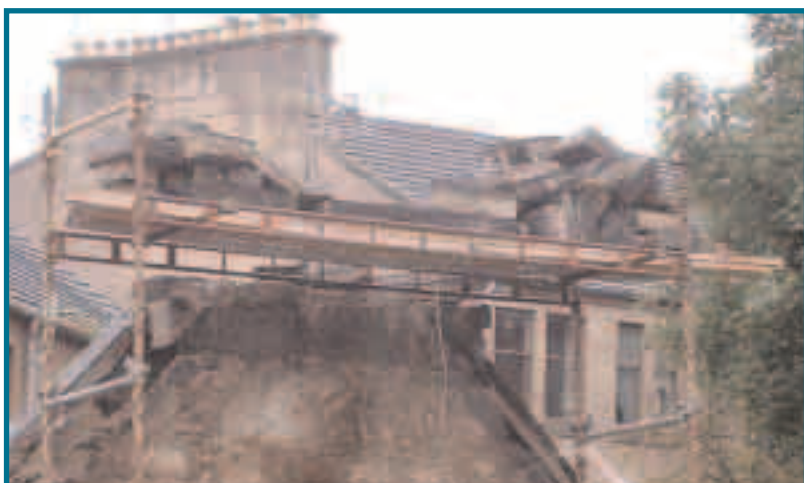
Five of the worst (from top clockwise) An accident waiting to happen, how not to work at height, an unsafe work platform, scaffolding resting on bricks, an unsafe support for scaffolding.
