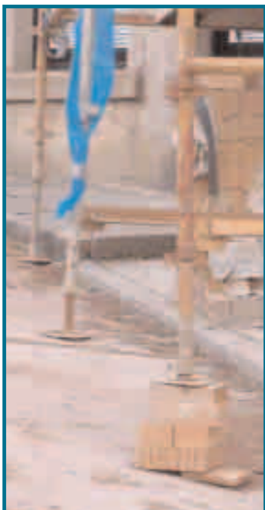
Five of the worst (from top clockwise) An accident waiting to happen, how not to work at height, an unsafe work platform, scaffolding resting on bricks, an unsafe support for scaffolding.
