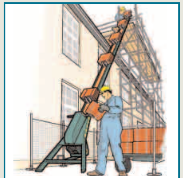
An inclined hoist in operation
