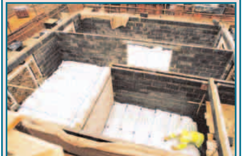
George Wimpey UK use a beanbag fall arrest system
