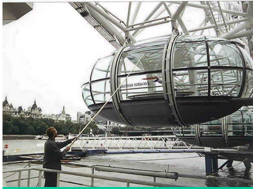
Windows being cleaned from the ground rather than off ladders
