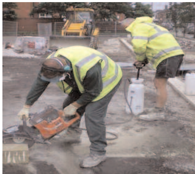
Figure 1 Use of water suppression to effectively control dust
